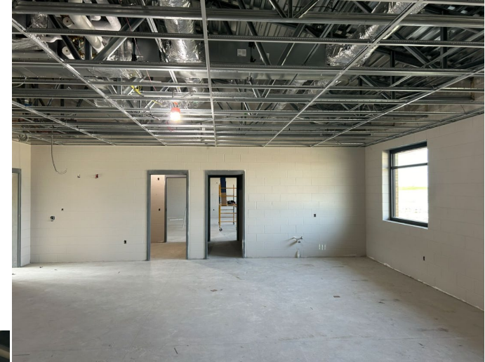
Classroom Ceiling and Painting
