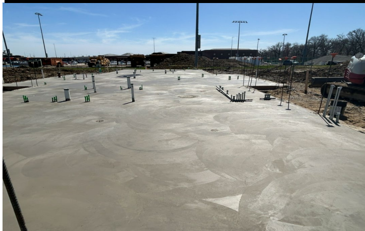
Community Building Concrete Slab
