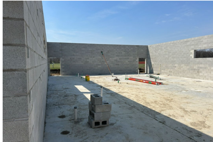
North Star Building CMU Walls
