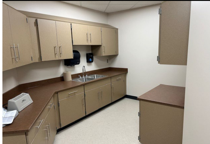
Cabinets & Sink in Admin Workroom
